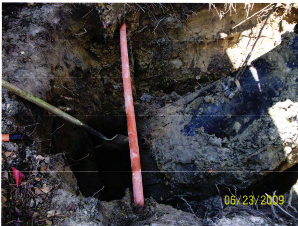
Picture 2: UST 1144Iris-1 during removal.
