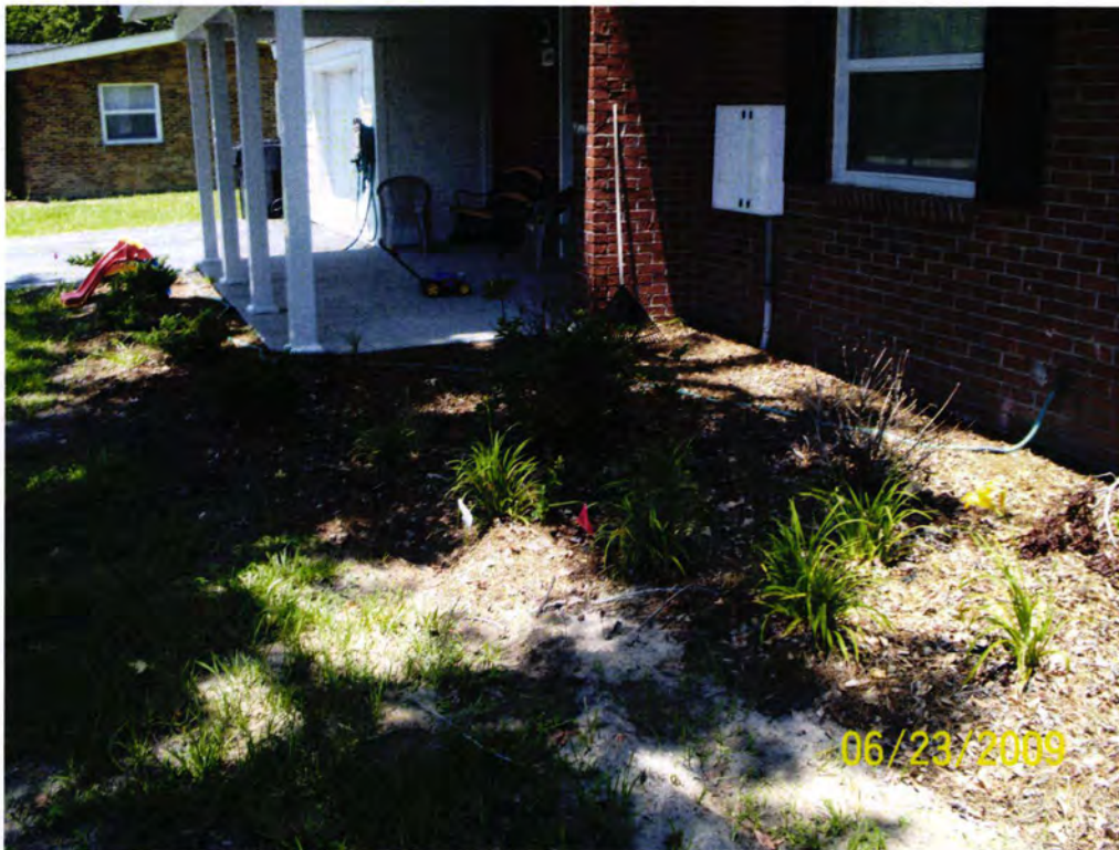
Picture 1: Location of USTs 1144Iris-1 and -2 before removal.
